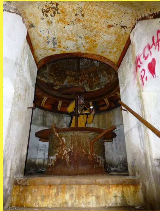
Werk 52 1/2S Skotinki - Panzerstand S58 für 8cm Panzerkanone M94 armoured coupola S58 for a 8cm canon M94
